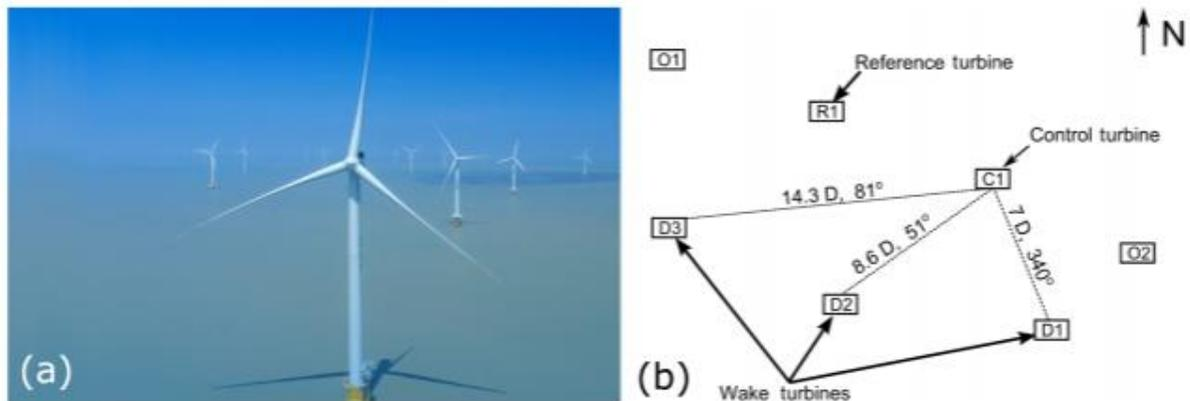
Figure 1: (a) Rudong wind farm used in the field study. (b) Turbine locations. The wake-steering control strategy is implemented to mitigate the wake interactions between C1, on the one hand, and D1, D2, and D3, on the other. As indicated by the diagram, C1 is the control turbine, R1 is the reference
